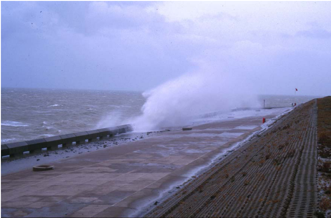
Figure 6 Example of overtopping rate of about 0.3 l/m/s at Samphire Hoe (photo HR Wallingford)
