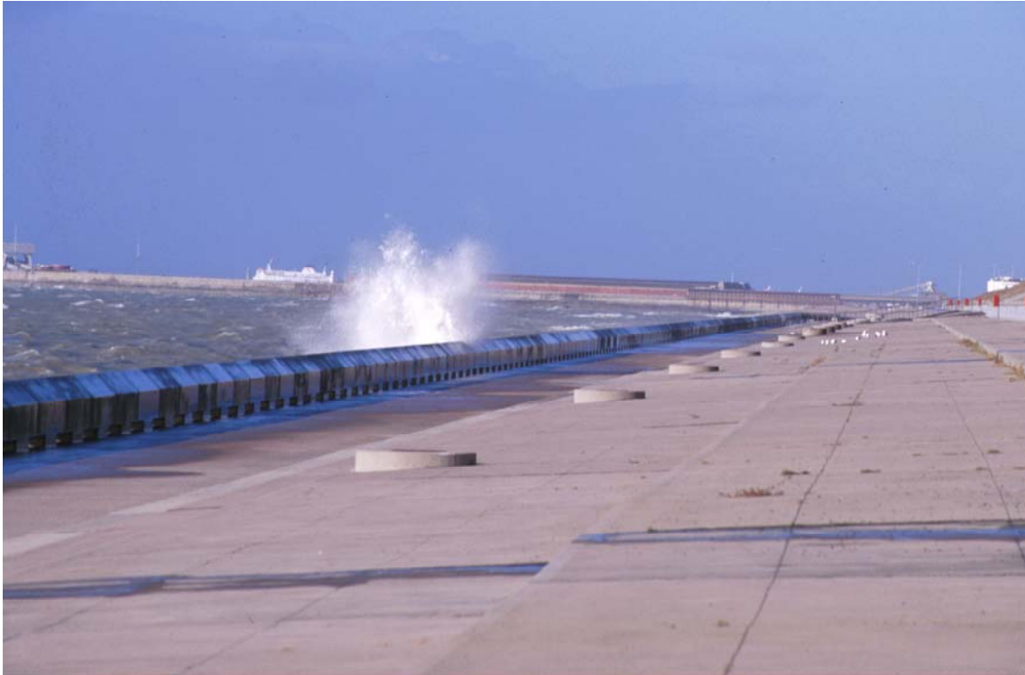
Figure 5 Example of mean overtopping rate of about 0.03 l/m/s at Samphire Hoe (photo HR Wallingford)
