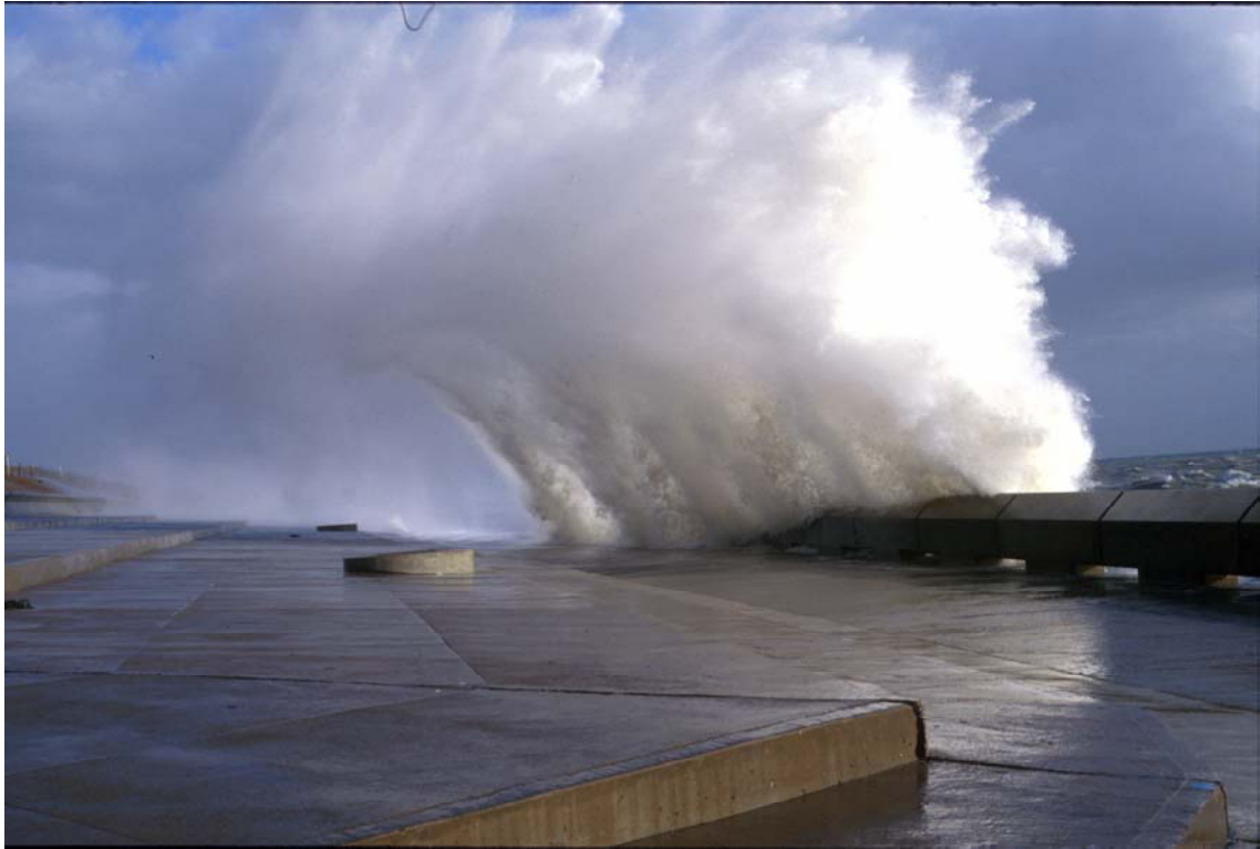
Figure 7 Example of peak overtopping occurring during mean overtopping rate of about 3.0 l/m/s at Samphire Hoe (photo HR Wallingford)
