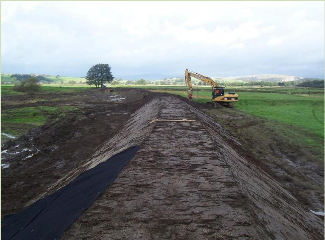
**Figure 2: Set back flood embankment during construction, looking upstream**
