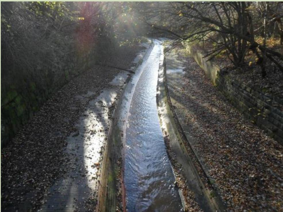
**Figure 1: Uniform brick-lined channel of the Medlock**
