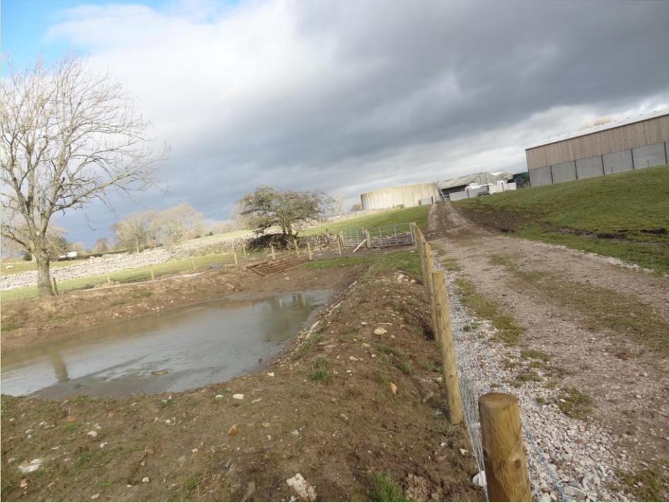
**Figure 2: Sediment trap in the Morland catchment**
