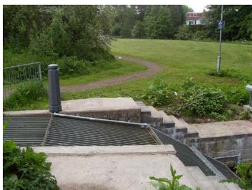
**Figure 1.1 Example telemetry and level sensor set up at a trash screen**
