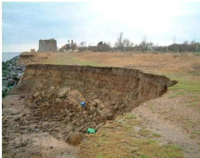
**Figure 1.2 Erosion of Environment Agency flood defence embankment, November 2004 (source: Terry Oakes Associates Limited)**
